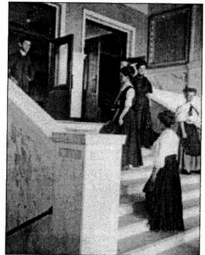
Workers entered the Administration Building through the marble-clad lobby, which remains today. Its elegance indicated the company's desire to provide attractive surroundings for its employees, as well as concern for corporate appearance beyond the utilitarian.
